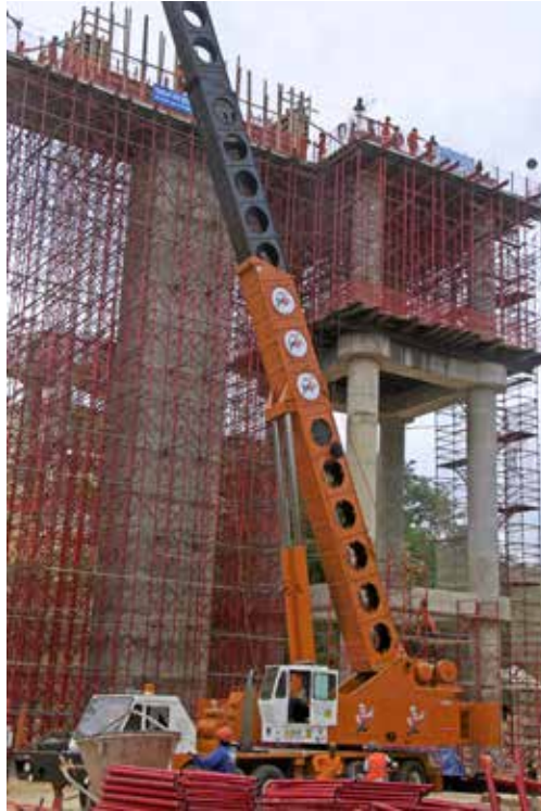
Concrete support columns for the bridge over Río Dulce.
